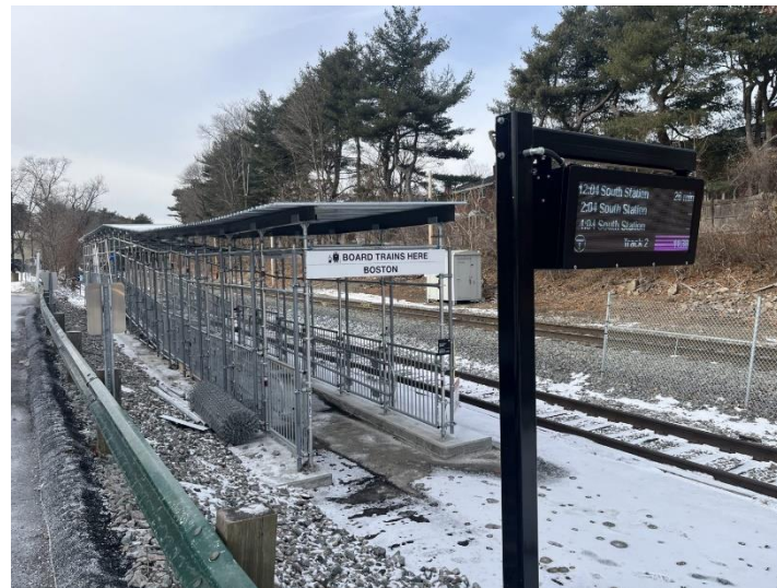
Figure 6: Images of two new ADA-compliant Mini-High Platforms at Wellesley Square Station. The entire project, including other upgrades, cost $3 million.
