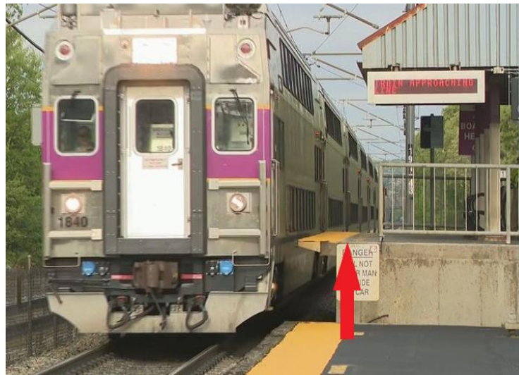
Figure 5: An example of raised platform that provides pedestrians with easier access to the train at entrance level, compared to ground level.
