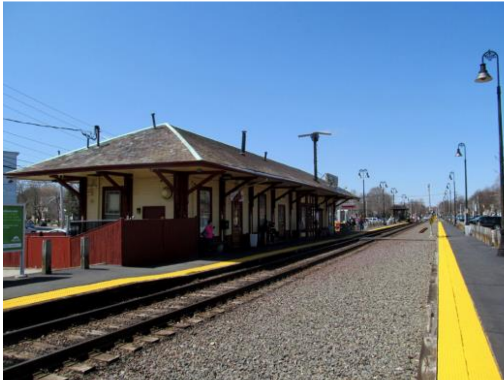
Figure 3: Current Reading Station looking northwest. Ample space is available for a second track on the northeast side of the existing track.
