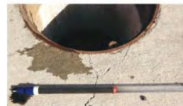
Inspection Utilitizing Sediment Probe
