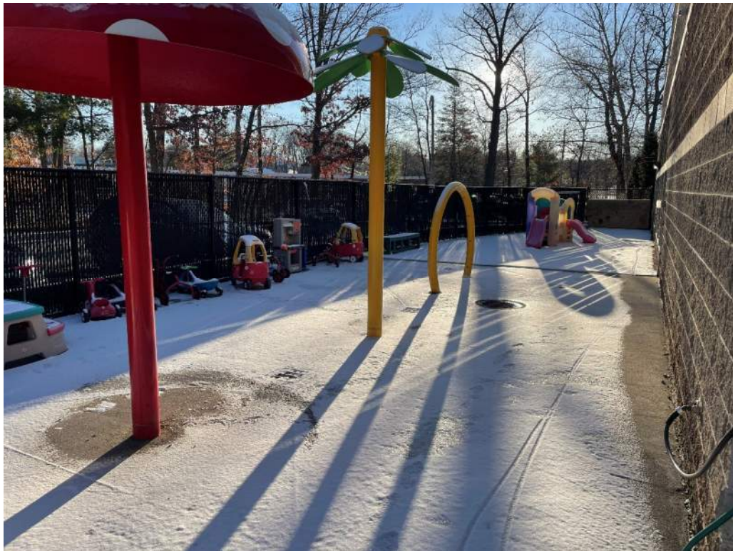
Photo 4: Existing Splash Pad & Synthetic Play Area
