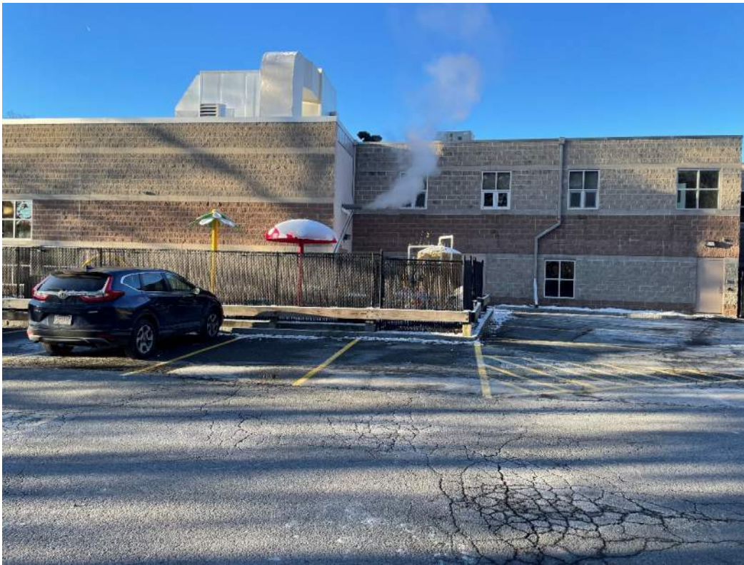
Photo 2: Existing Fence Enclosure/Concrete Splash Pad
