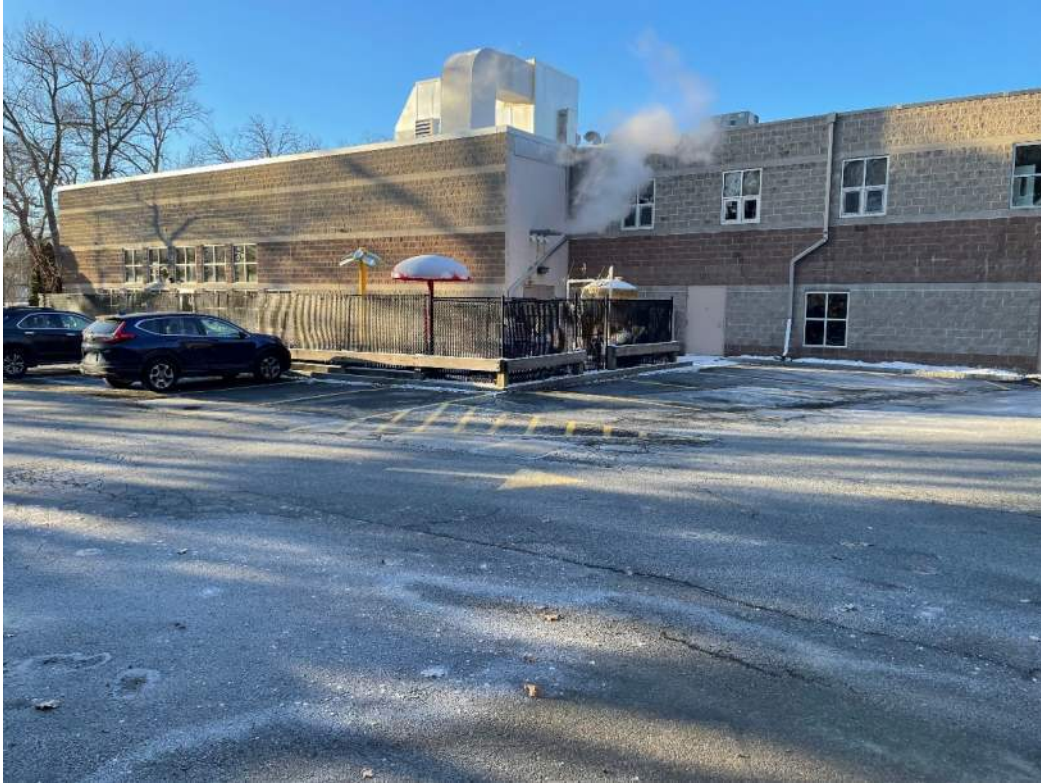
Photo 3: Existing Fence Enclosure/Concrete Splash Pad Area
