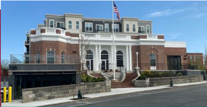
8 Sanborn Street- Post Office (2021-22)
