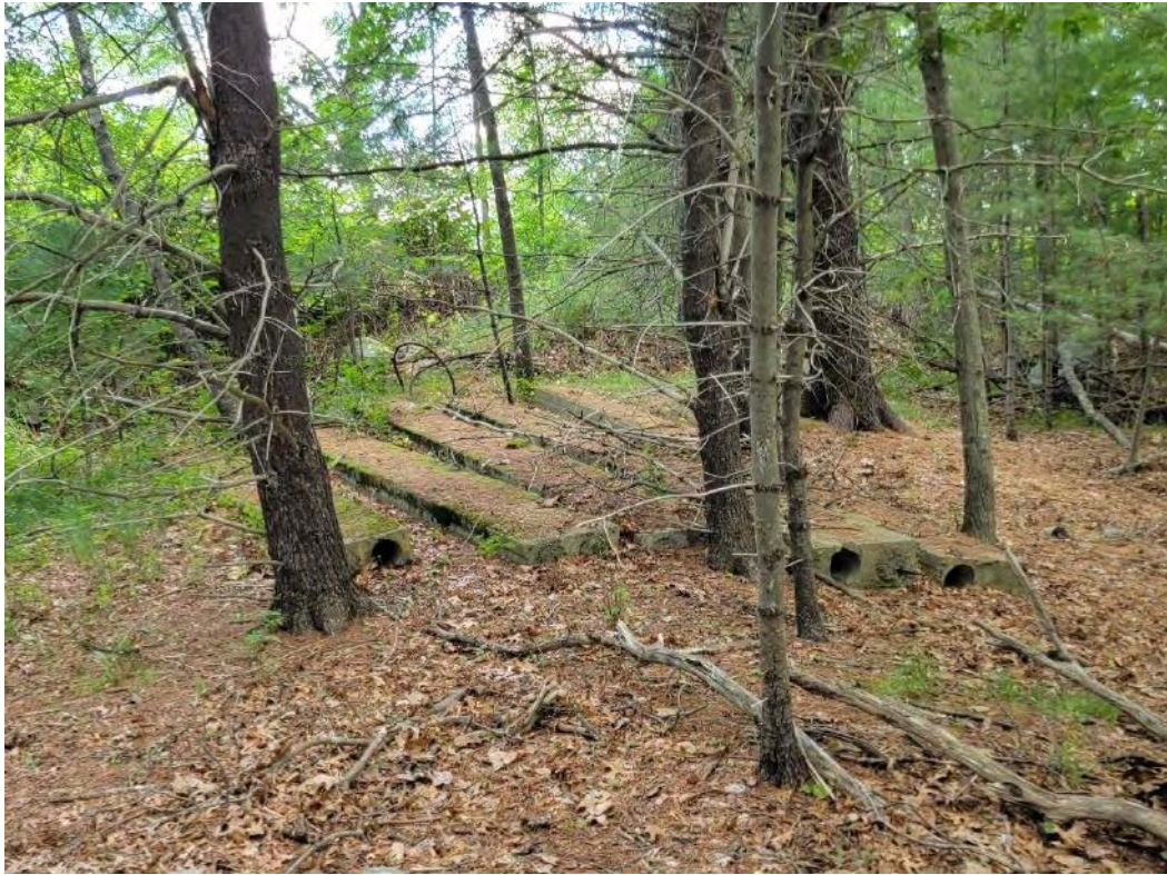
Photo 5: Concrete post tension slabs between TP- 103 and TP-107.
