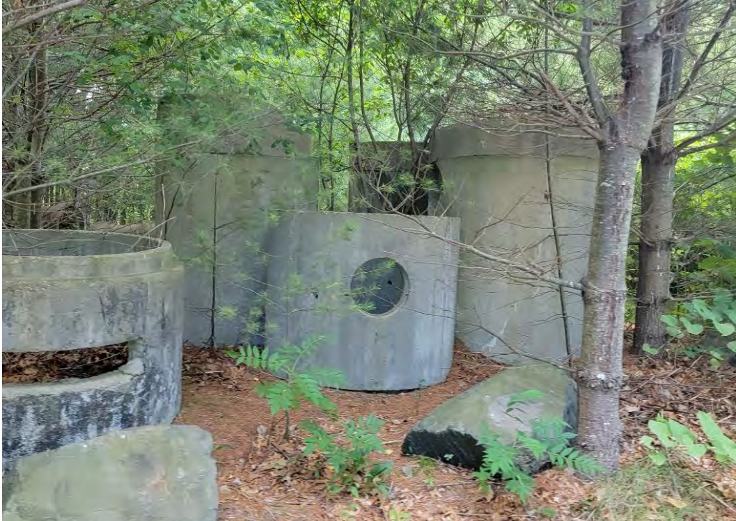
Photo 3: Precast concrete manhole structures between TP-105 and TP-106 close to the road.
