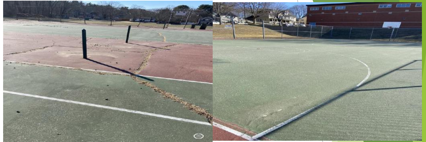
Existing conditions at Barrows
